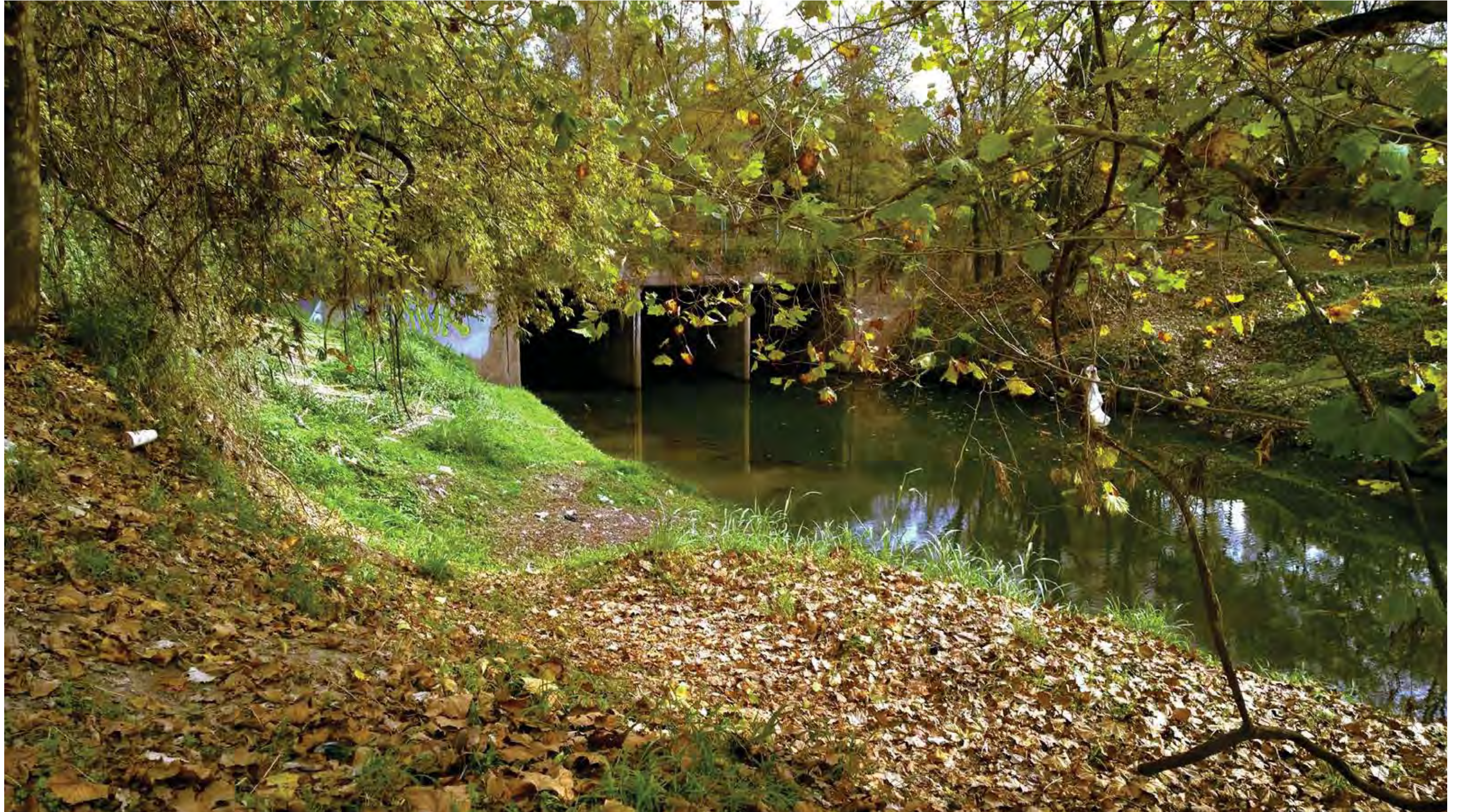
(RIGHT): Existing Trail at Eastern Lawn South of Community Center; (TOP): TXDOT Outfall Little White Oak Bayou
